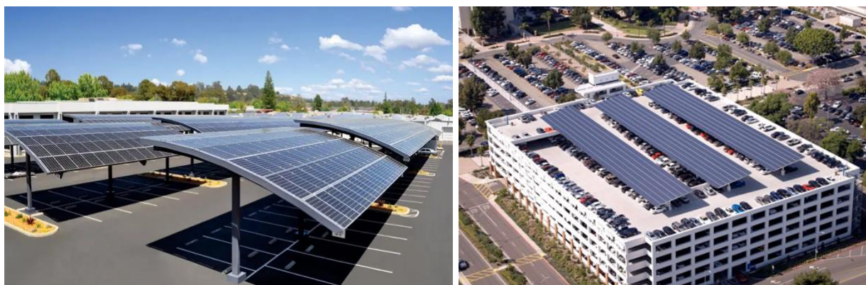
Exhibit 51: Example of a solar car canopy built in a parking lot and a parking structure. Source: Friday LLC
